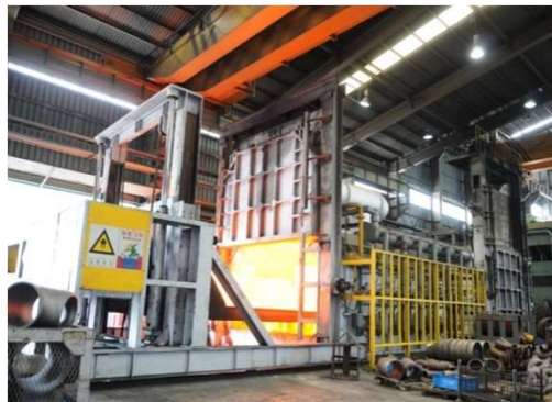
Heat Treatment Furnace For Fitting
